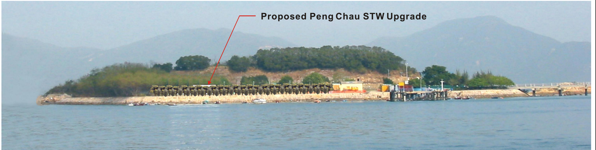
Future View from South of Tai Lei Island with Landscape Treatment at year 10 of the operation stage
