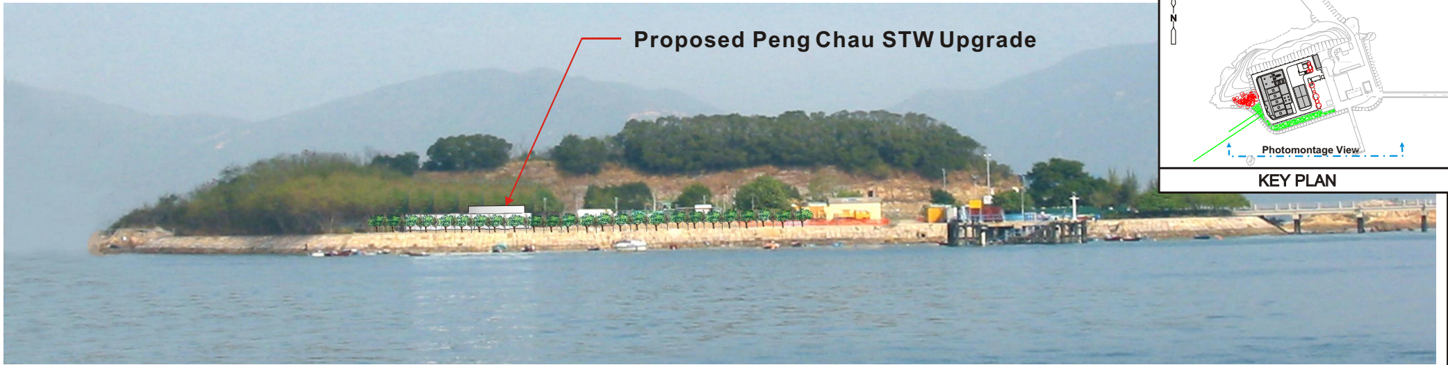
Future View from South of Tai Lei Island with Landscape Treatment at day 1 of the operation stage
